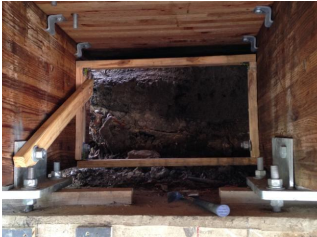
Back wall panels are installed at the abutments between each girder.
