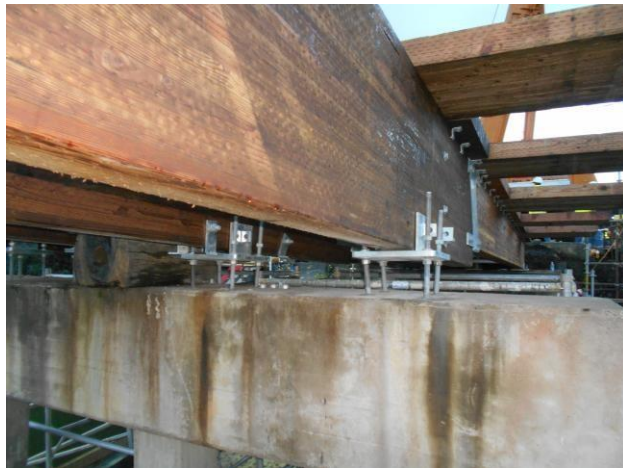
The glulam girders are anchored to the concrete caps using specially fabricated jack-posts.
