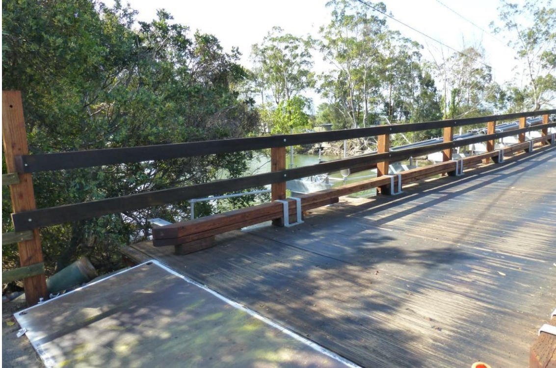
Finished kerb and approach.
