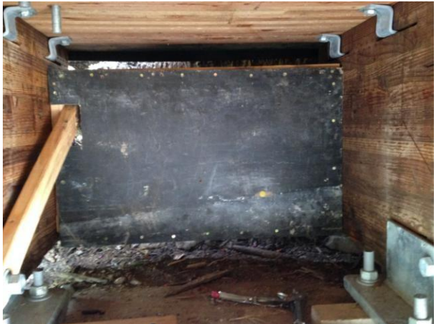
Back wall panels are installed at the abutments between each girder.
