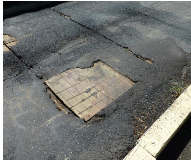
The asphalt running surface is showing signs of wear, and has completely come away from the underlying plywood deck in places.
