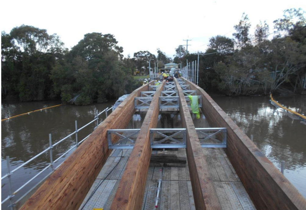
Glulam girders completely installed.
