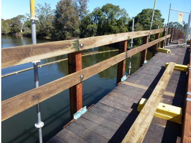
A new timber guard-rail system is installed (left photo). The guardrails are braced using steel cross-bracing running from the guardrail post to the bottom of the adjacent deck panel (right photo).
