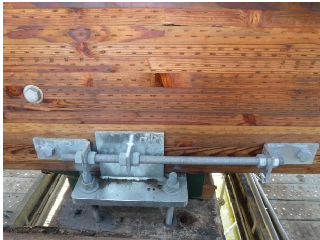
The glulam girders are anchored to the concrete caps using specially fabricated jack-posts.
