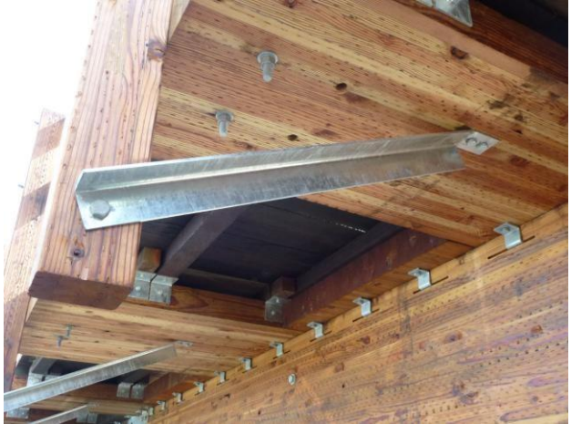
A new timber guard-rail system is installed (left photo). The guardrails are braced using steel cross-bracing running from the guardrail post to the bottom of the adjacent deck panel (right photo).
