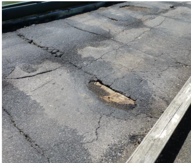
The asphalt running surface is showing signs of wear, and has completely come away from the underlying plywood deck in places.
