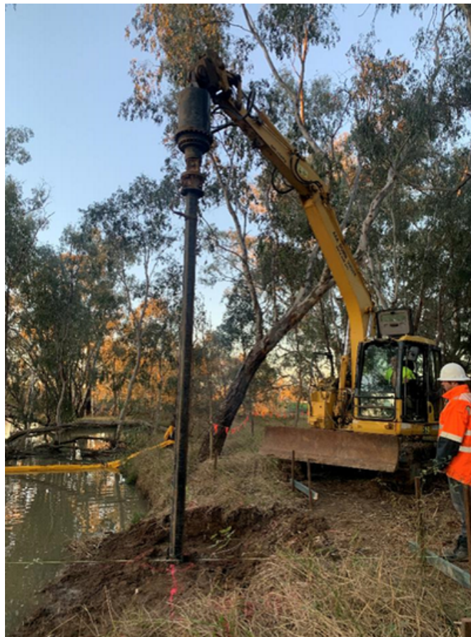
TRS crews screw piling along banks
