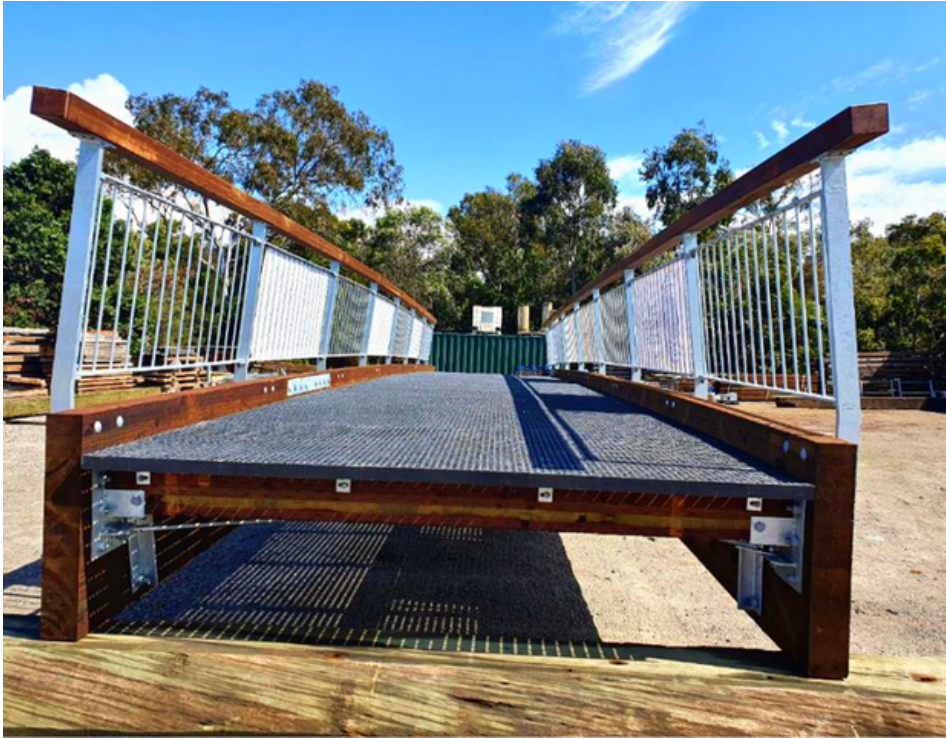
Treated Engineered Glulam Side Girders with FRP mesh grating.
