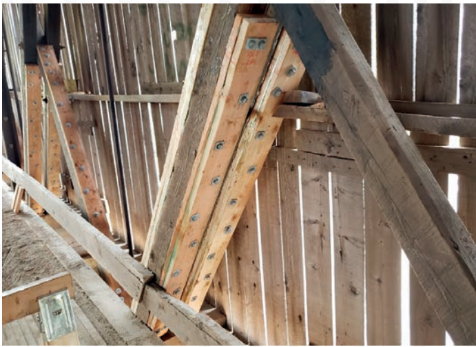
Photos above and to the right shows Retrocom® Reinforcement installed onto trusses
