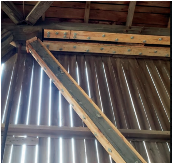
Photos above and to the right shows Retrocom® Reinforcement installed onto trusses
