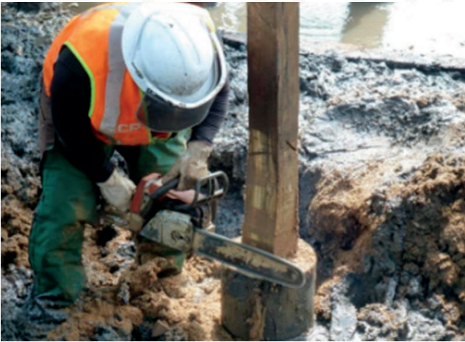
Above the technician squares up the affected pile
