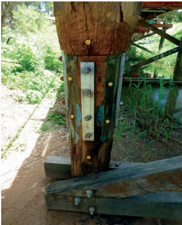
Photo to the left: Pile posting completed with rotation spline and steel side plate. Note yellow diffuser plugs indicating where the diffuser rods have been placed once the piles were posted.
