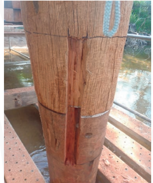
The pile shown above has been Taper cut for rotation spline slots. Photo below shows the application of structural epoxy (2 part paste, odourless, 100 percent solids), to the slots.
