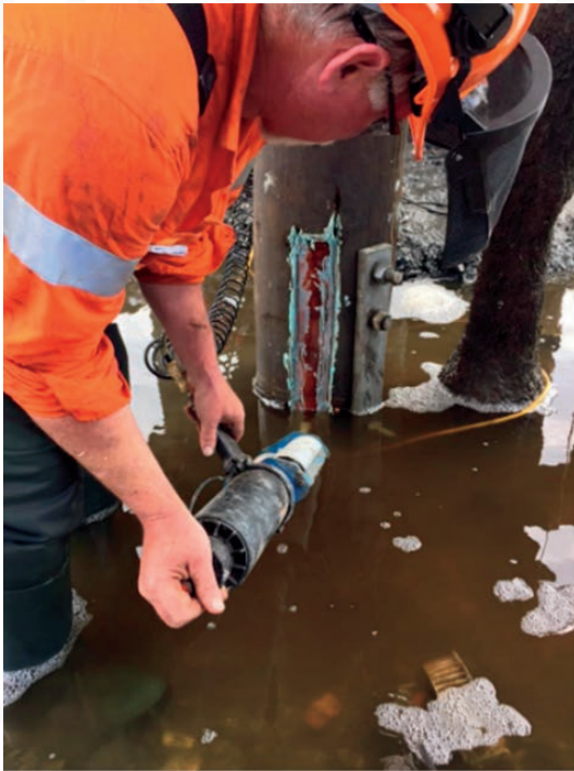
Injecting a pile cavity with Structurfill® Epoxy once wrap is in place and cured
