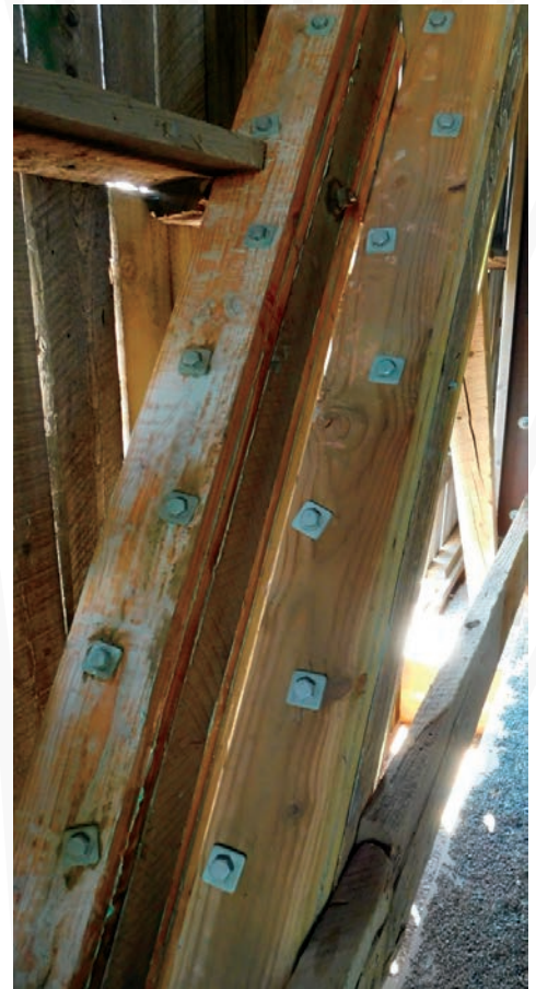
Retrocom® Reinforcement installed on two sides of the trusses and onto the beams above
