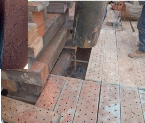
The pile shown above has been Taper cut for rotation spline slots. Photo below shows the application of structural epoxy (2 part paste, odourless, 100 percent solids), to the slots.
