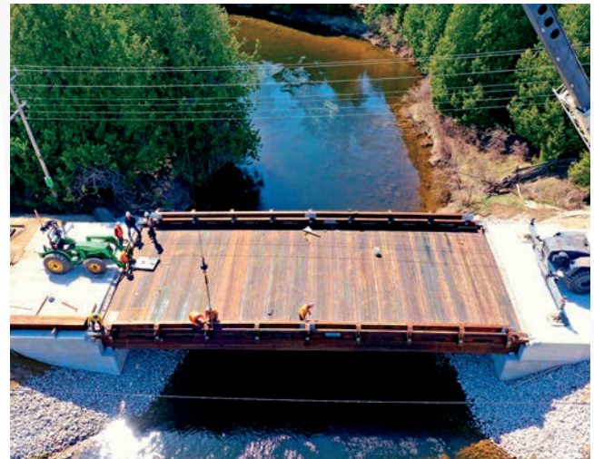
Lantz Bridge - Installation
