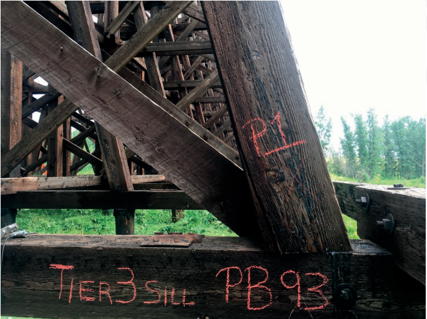
Tier 3 Sill, Pile Bent 93, Pile 1
