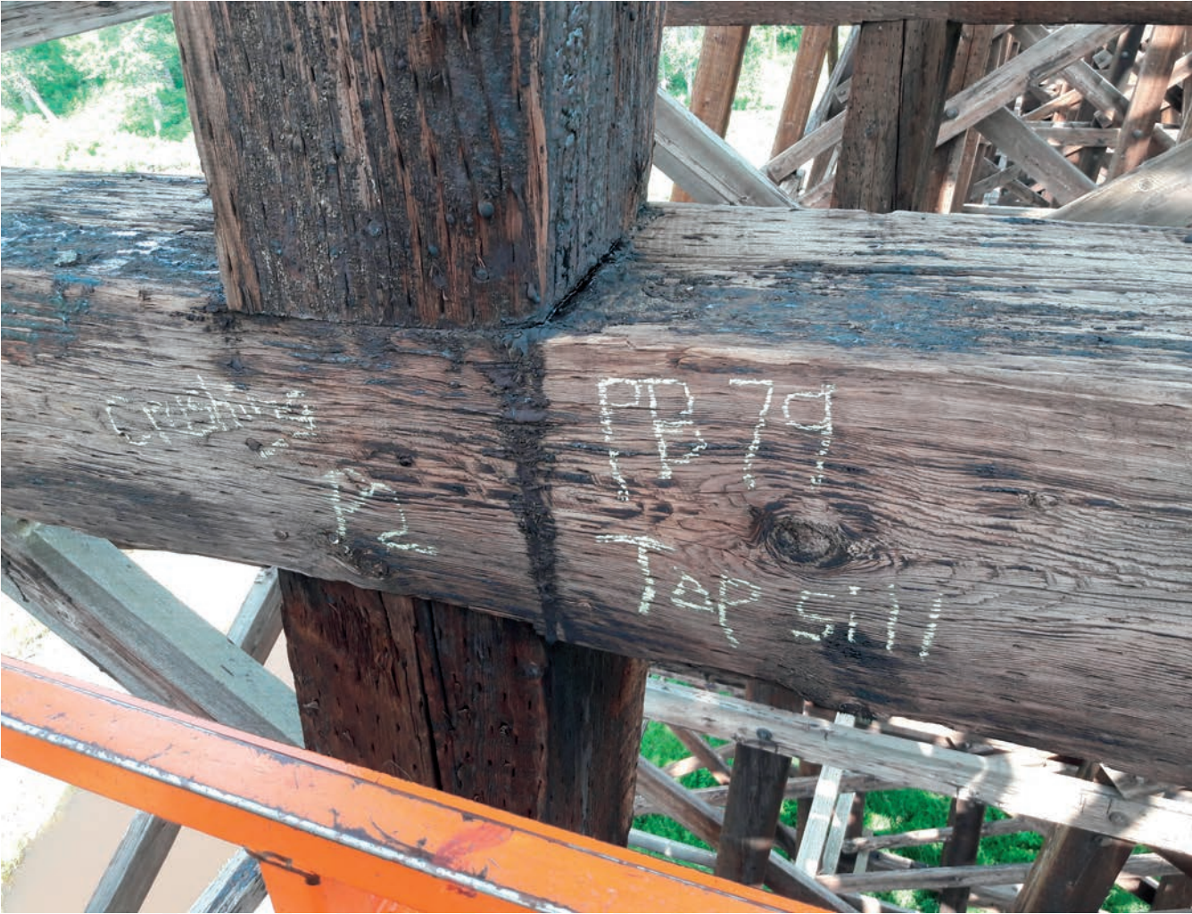
Top Sill, Pile Bent 79, Pile 2
