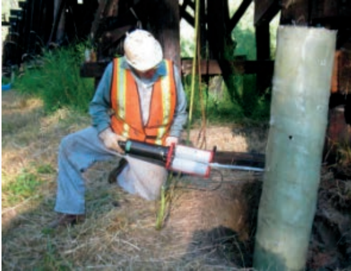
Injecting a pile cavity with Structurfill® Epoxy once wrap is in place and cured
