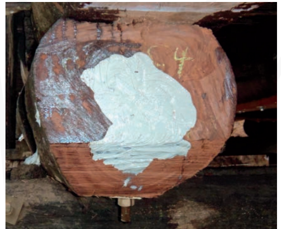
Cross section view of structurfilled pile
