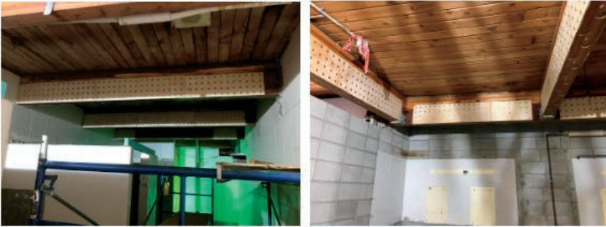
Above Shear panels installed in an Aquatic Center in Camrose, Alberta.
