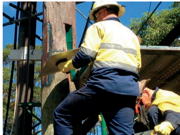
Photo to the left: Pile posting completed with rotation spline and steel side plate. Note yellow diffuser plugs indicating where the diffuser rods have been placed once the piles were posted.
