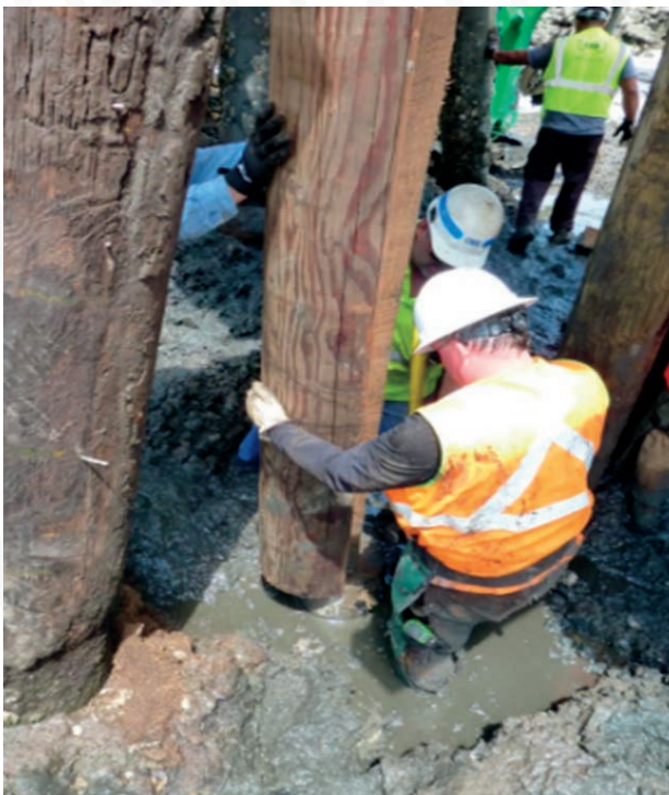
The two halves are installed one at a time, then glued and screwed together. After installation is complete the the interior will receive two part, slow cure, 90 mpa Structurfill® Epoxy
