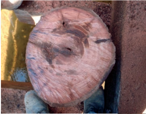
The pile shown above has been cut to good wood
